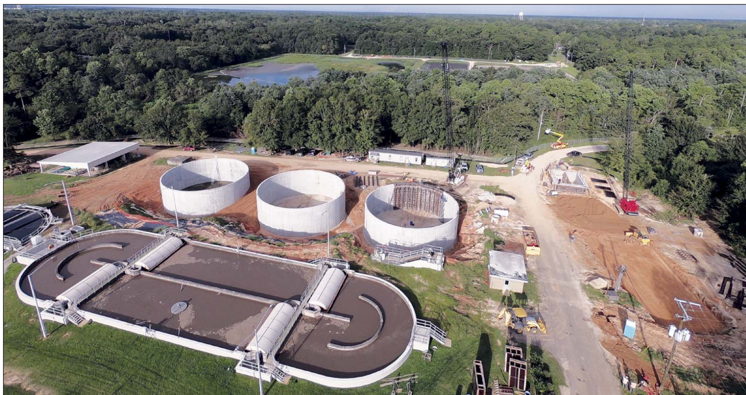
Figure 9. Wolf Creek Wastewater Treatment Plant Construction, September 2018 (courtesy of Goodwyn, Mills & Cawood)
